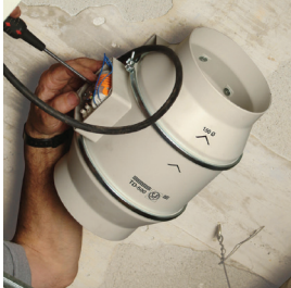
Carry out the wiring connections.
