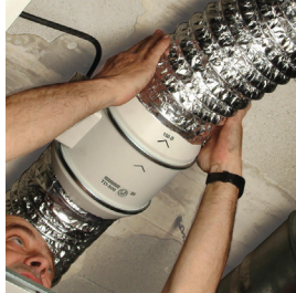
Connect the ducts.
