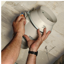
Place the impeller and motor assembly.
